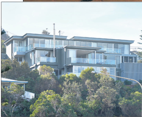
LOFTY: The three-storey Killcare Beach House.
